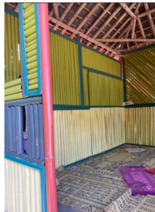
Fig. 4. Outside (a); and inside (b) views of the mushola wall made from ampel ( Bambusa vulgaris subspecies) bamboo
