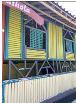
Fig. 4. Outside (a); and inside (b) views of the mushola wall made from ampel ( Bambusa vulgaris subspecies) bamboo
