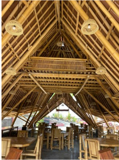
Fig. 3. The roof truss, lamp shade, tables and chairs are fully made from Ampel ( Bambusa vulgaris subspecies) bamboo
