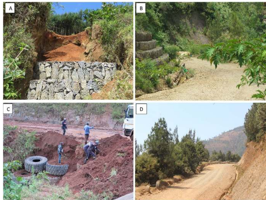
Figure 2. Gabion baskets in support of the main access road (A) and a wall side (B); tires being positioned to support an access road with drainage (C) and concrete side drains on the wall side (D).
