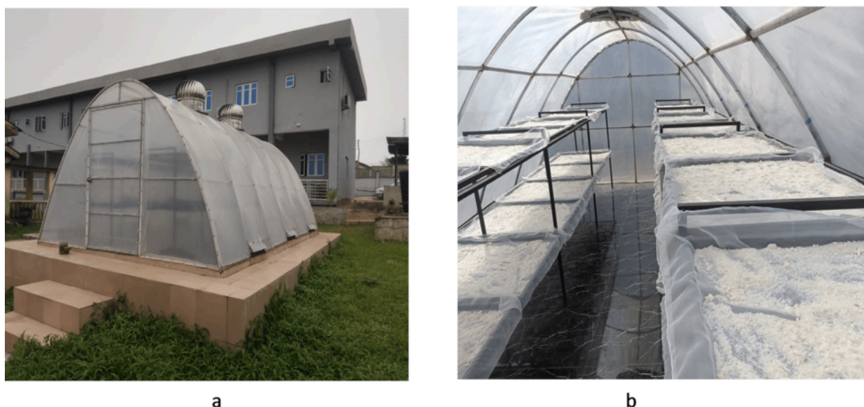
FIGURE 2: (a) Exterior view of NSPRI PSSD installed at Ibadan Zonal Office; (b) Interior view of the drying chamber during the evaluation
