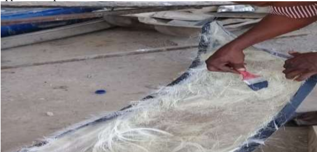
Plate IX: Application of polyester- resin to the fibre
