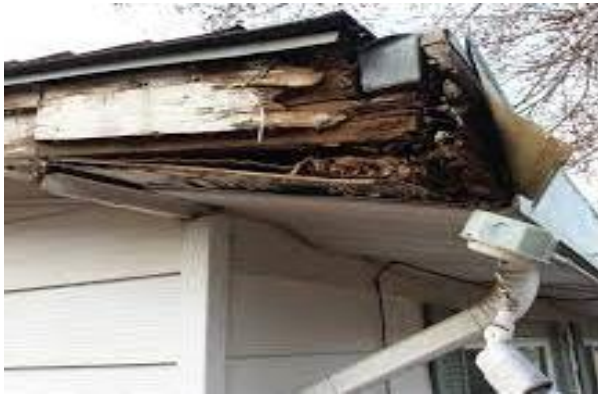
Plate 7A: Effect of fungal on facial board substrate
