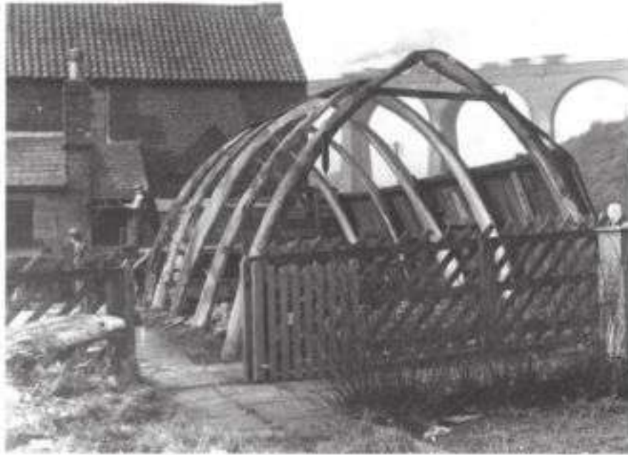
Figure 2. Storage shed in the process of being dismantled, revealing its construction consisting of the paired jawbones of seven large baleen whales. It was situated close to the railway viaduct (N28909) in Whitby (Photo by Frank Meadow Sutcliffe. This image is reproduced from a print in the C.I. Massey archive.)
