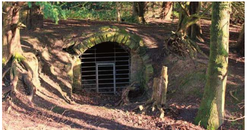
Plate 4 (see p33). 4a. Rockley Tunnel today.
