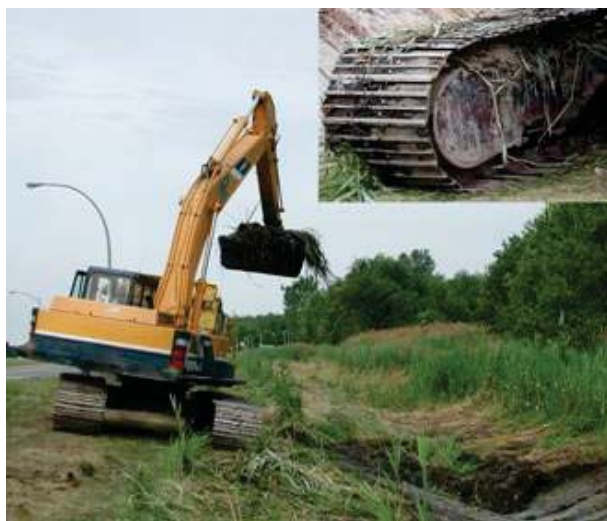
Figure 12. The Phragmites rhizomes in the soil from this ditch expansion operation will be dumped in a new location, but in addition the rhizomes attached to the track runner of this 360 excavator (inset – upper right) may be dislodged at the next work site, or along the way, giving rise to new stands. Photo by P.M. Catling in southwestern Quebec in 2005.
