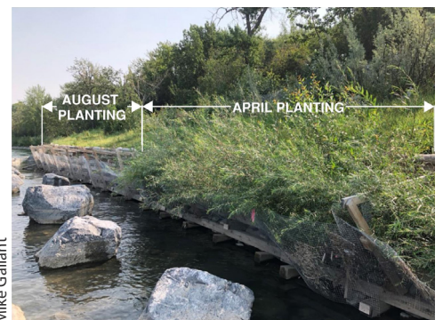
Successful establishment of live cuttings planted in April (right side of timber cribwall) and failure of live cuttings planted in August (left side of timber cribwall) ♦
