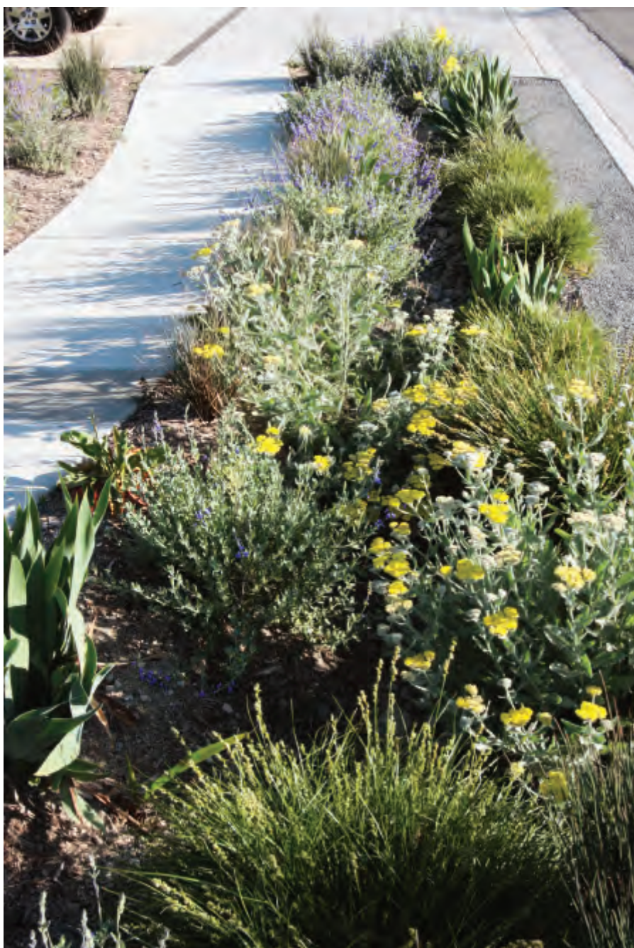
Elmer Avenue vegetated swale with maturing plants veiling the gravel-lined swale on a sunny day. Sanddune sedge ( Carex pansa ), spreading rush ( Juncus patens ), Germander sage ( Salvia chamaedryoides ), moonshine yarrow ( Achillea 'Moonshine'), bearded iris ( Iris sp.).
