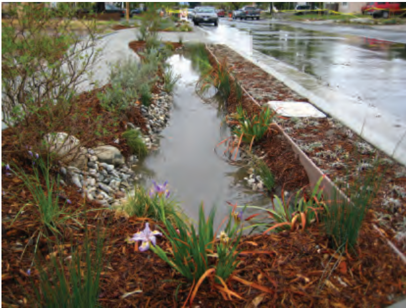
Rock and gravel-lined swale on Elmer Avenue fills up with stormwater on a rainy day. Note the meandering sidewalk and dymondia ( Dymondia margaretae ) in the 18" next to the curb for passengers exiting cars. The landscaped area includes Douglas iris ( Iris douglasiana ), spreading rush ( Juncus patens ), sanddune sedge ( Carex pansa ), autumn sage ( Salvia greggii ), and germander sage ( Salvia chamaedryoides ).
