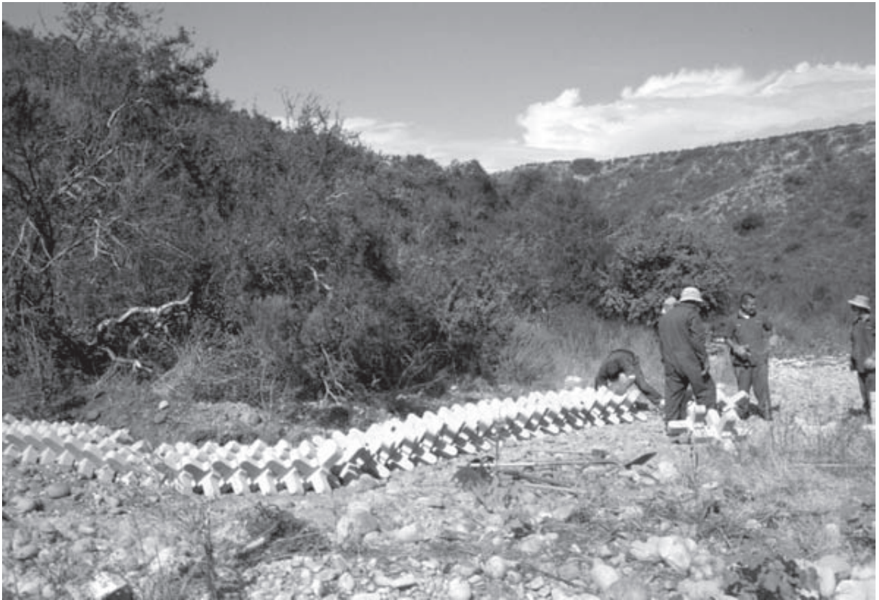
A-Jacks, erosion control devices in Lopez Canyon, San Diego County, used to check water flow and thus protect the habitat of the rare willowy monardella. All images used courtesy of City of San Diego, 2003.
