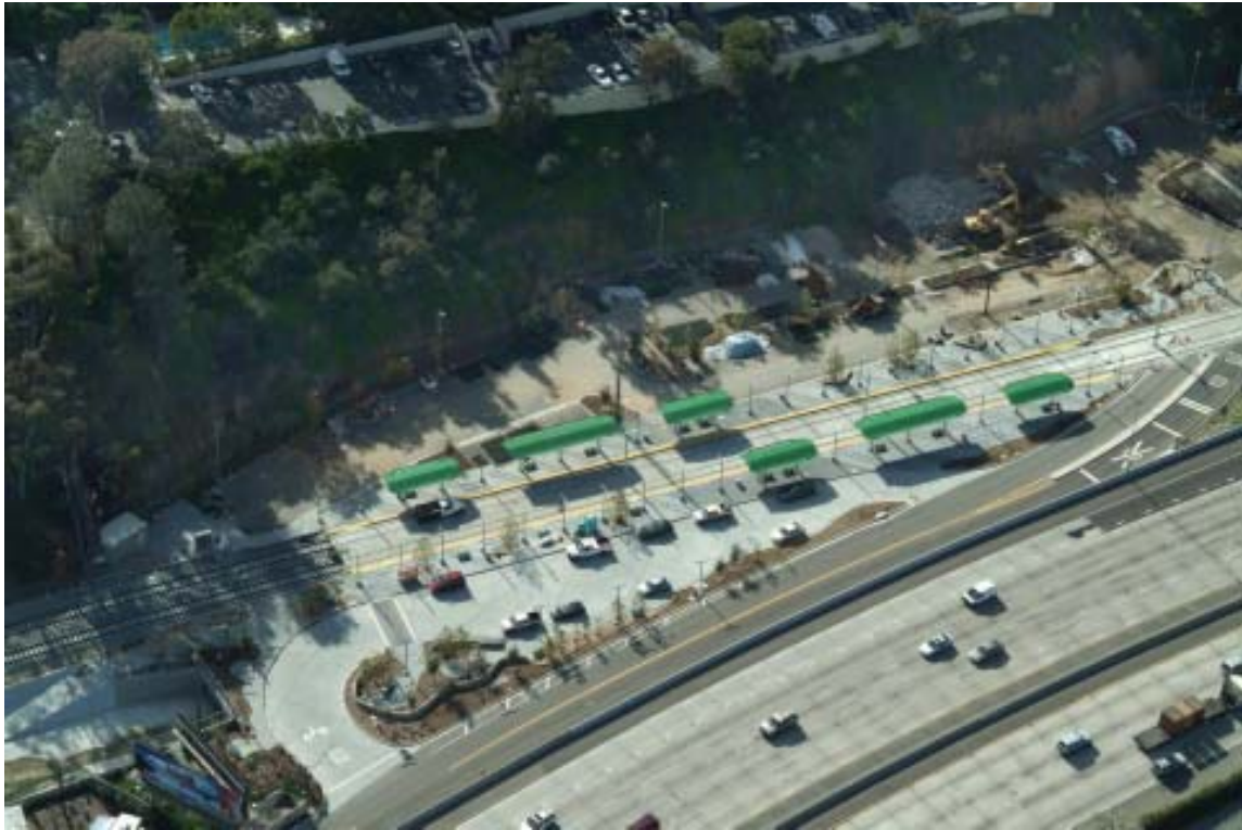
Aerial view of the 70th Street trolley station during construction.
