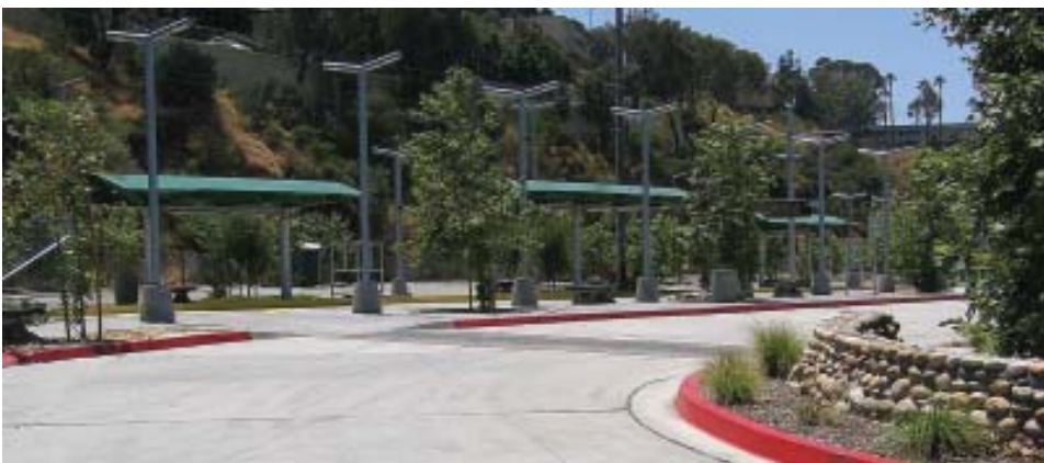
Overview of the 70th Street trolley station.
