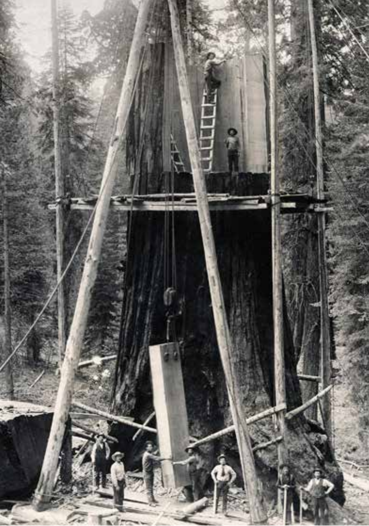
Figure 6. An 1892 photo of workers dismantling the General Noble Tree to create a two-story building for the 1893 World Columbia Exhibition. [C.C. Curtis, California History Section Picture Catalog: California State Library.]
