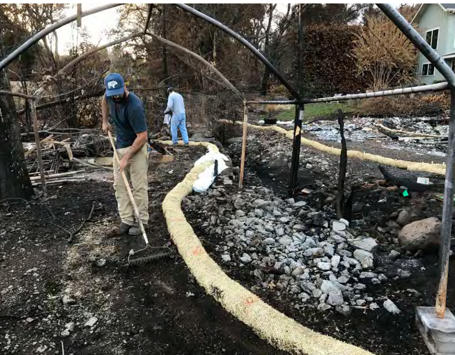
Sonoma Ecology Center staff and volunteers install fiber wattles to prevent toxic materials and erosion from burned homesites reaching local creeks.
