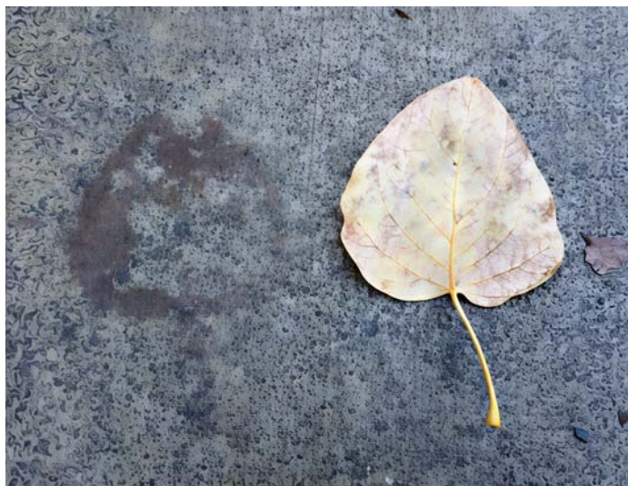
Concrete sidewalk stained by black cottonwood leaf. PHOTO: ERIC WORDEN
