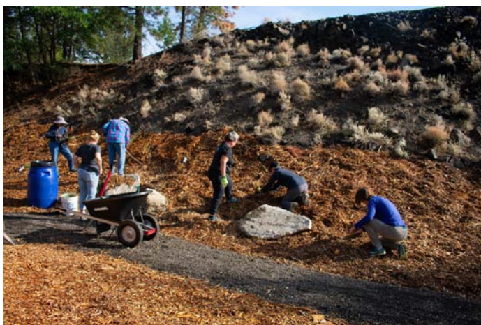
Project volunteers work together to install native plants. PHOTO: THURMAN JOHNSON
