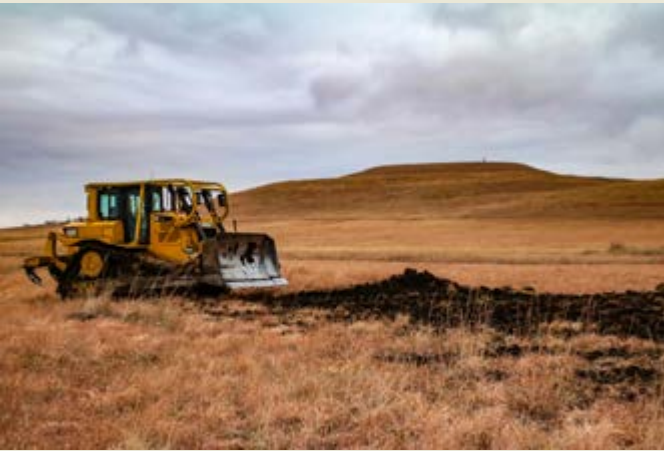
Doug Nihart, of Ebert Construction, begins leveling ten of the thirteen terraces.
