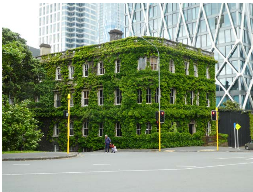
Fig. 1. Boston ivy covering the Northern Club building, 19 Princes St, central Auckland. Because of the adhesive disc-like tips on the short, but much-branched tendrils, the vine attaches firmly to rock or wood. Photo: 16 Nov 2021.
