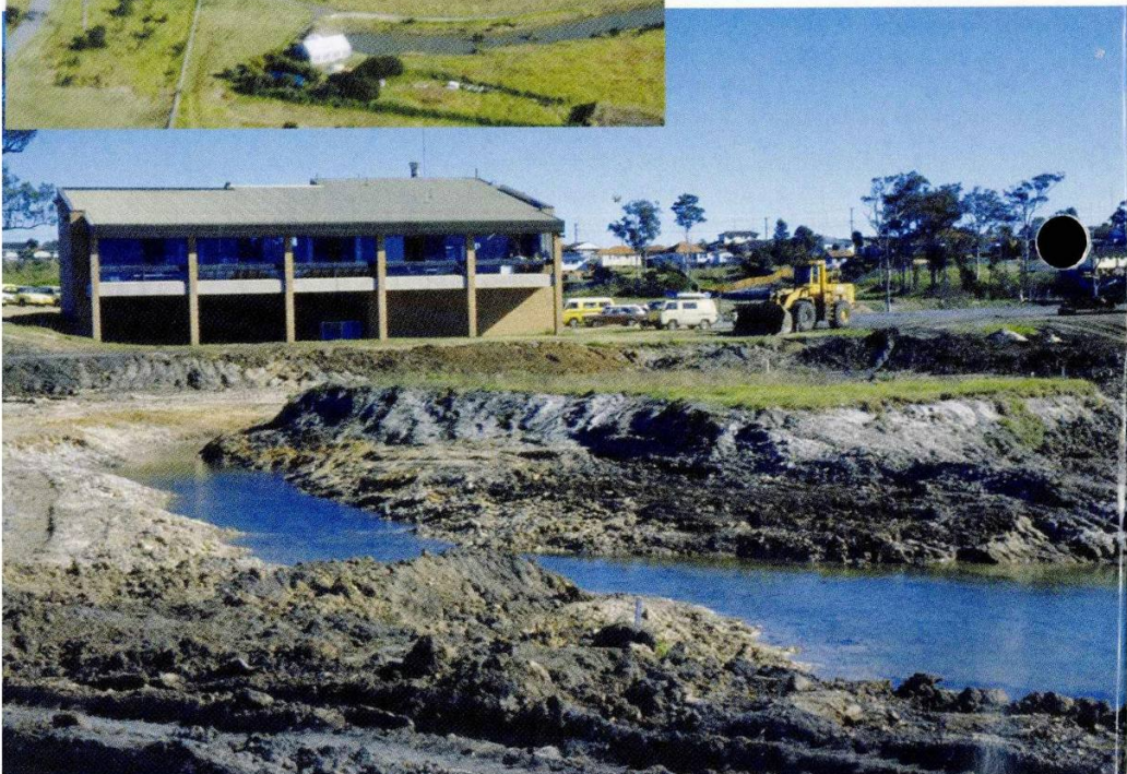
Below - Pond Excavation, June 1986 All photos on both pages Paddy Lightfoot
