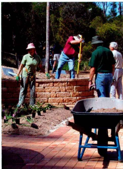
Volunteers enjoy the final stages of a new development -- the plant out.
