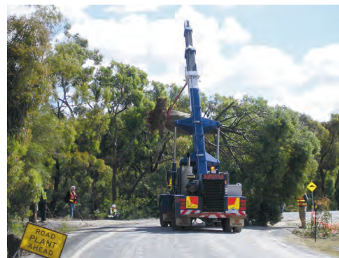
The heavy lift with the Bottle Tree finally out of the ground.
