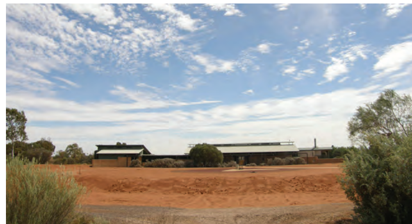
The forecourt of the Visitors' Center being prepared for replanting, February 2010.
