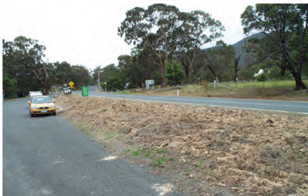
Site weeded, ripped and sprayed. All photos Jane and Phil Williams.
