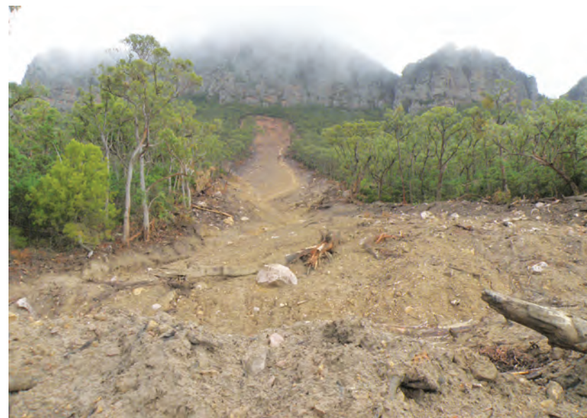
Landslip at Mt Abrupt
