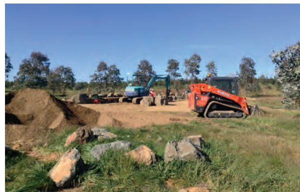
Constructing The Clearing
