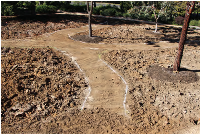
The new garden area dug over and the paths laid out
