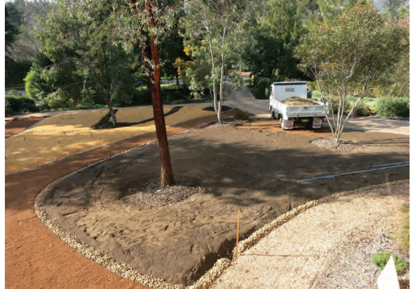
The last load of the new topsoil being delivered
