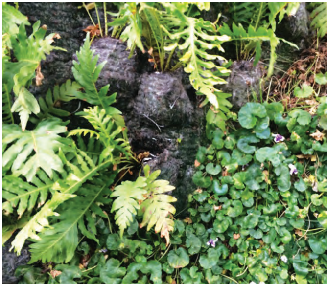
Some of the Australian native plants, growing on the vertical walls of One Central Park between two layers of geotextile matting. Photo: Mark Abell
