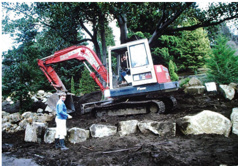
Sib Corbett directing proceedings during construction of the Tasmanian Native Section.
