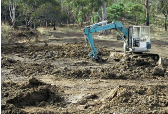
The excavator ripping up the deep dolerite clay.
