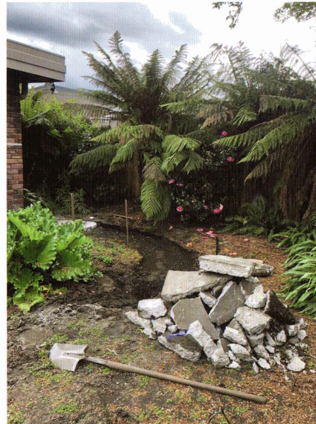
Preparing for a path through the garden by removing the old foundations of a Hills Hoist clothes line and path – 620kg of concrete!
