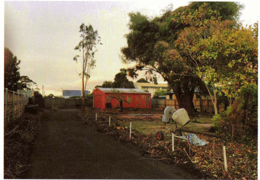
Removal of eastern hedge and much more by a professional arborist and which enabled us to set to work. Circa April 2019.
