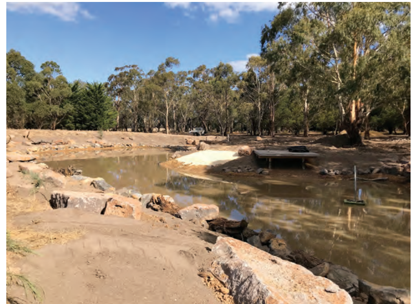
Paraparap dam construction. Emmaline Bowman.
