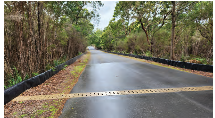
Driveway into RBGC showing tunnels. Miriam Ford.
