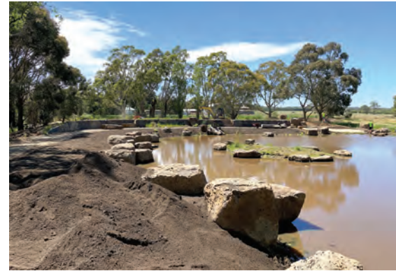
Kyneton construction. Emmaline Bowman.
