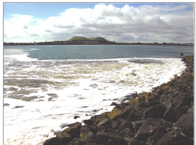
Fig. 17. Treated wastewater outfall, 1 May 2018.
