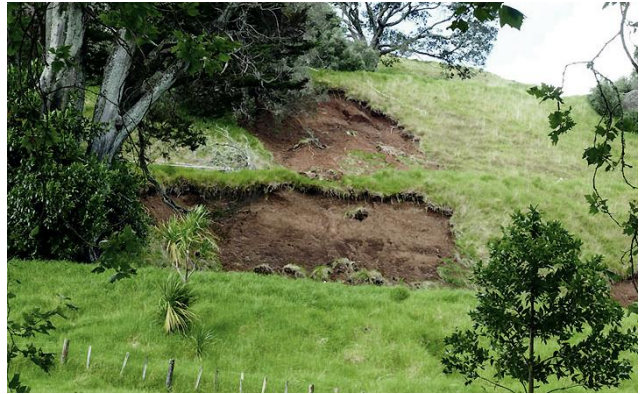
Fig. 2. Large recent slips on the northern slope of Maungakiekie. Photo: Philip Moll.
