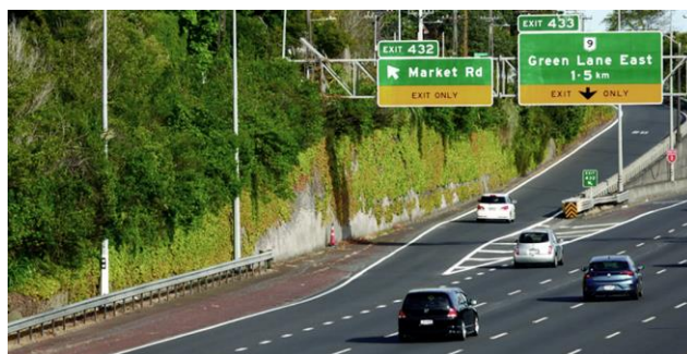
Fig. 7. Planted Boston ivy vines 450 m along concrete retaining wall, southern motorway, seen from Dilworth footbridge looking south towards the Market Road offramp Photo: SHD, 24 Oct 2022.
