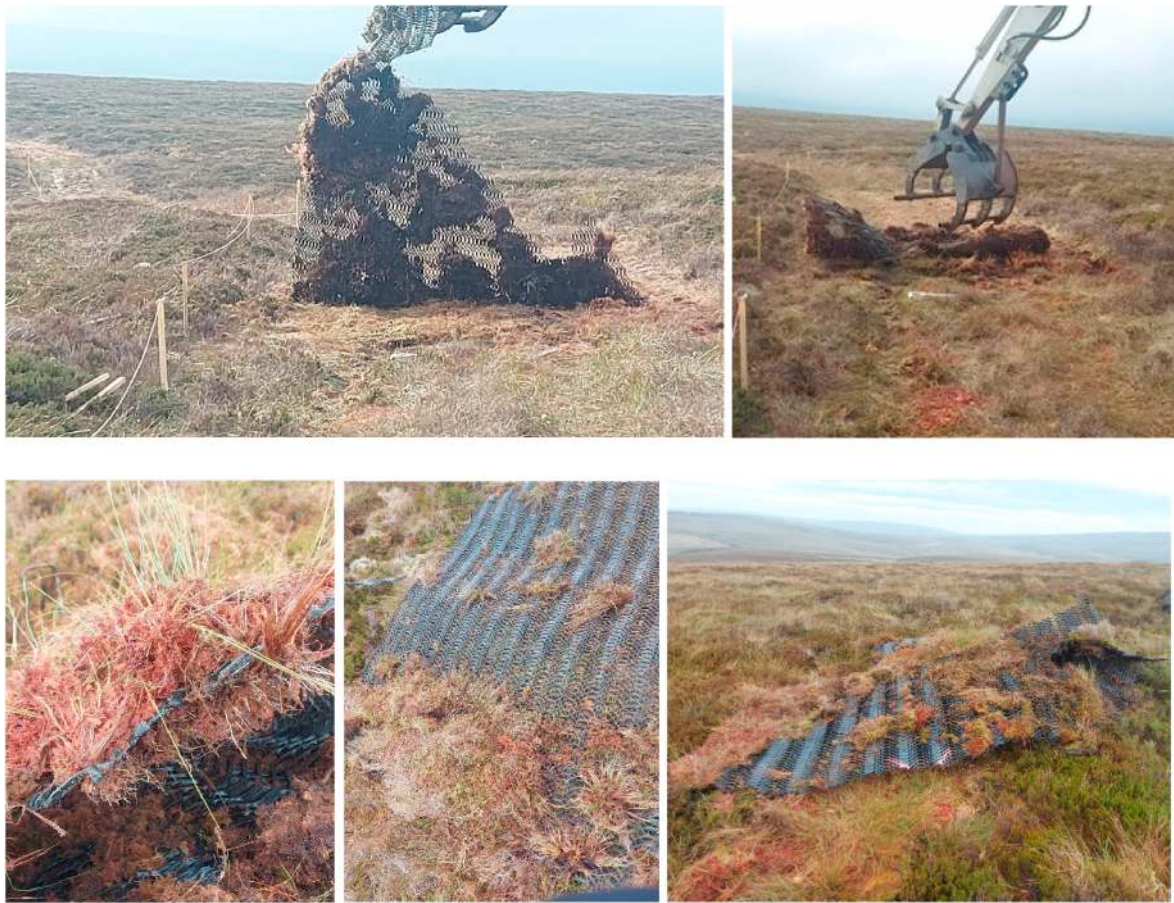
Fig. 2. Removal of sections of mesh track from the study site showing digger set-up and the extensive surficial vegetation loss that occurred during the removal process.
