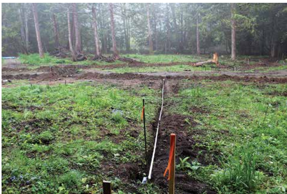
Fig. 5. Installing the irrigation system. Photo by Geoff Ball.
