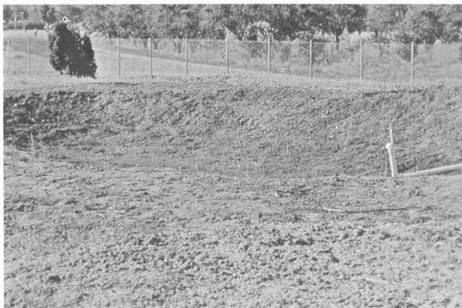
View of excavation for CP bog at the Fullerton Arboretum in September, 1979. The white pipe is the inlet for the RO water.
