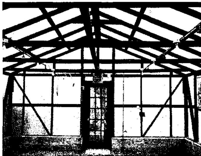
Inside house constructed of treated lumber and covered with "Corostron", a corrugated reinforced clear plastic material which comes in rolls of various widths. DR. W. F. MATHIS, Moultrie, Ga.
