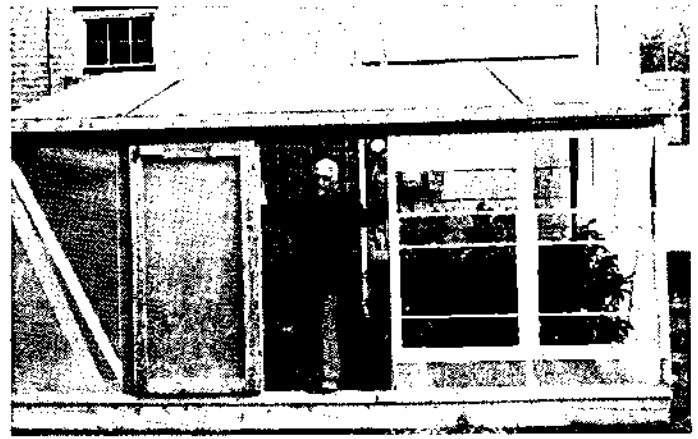
Lean-to polyethylene house with two storm windows for ventilation. Heated through basement door. N. Q. HANNER, Greensboro, N. C.
