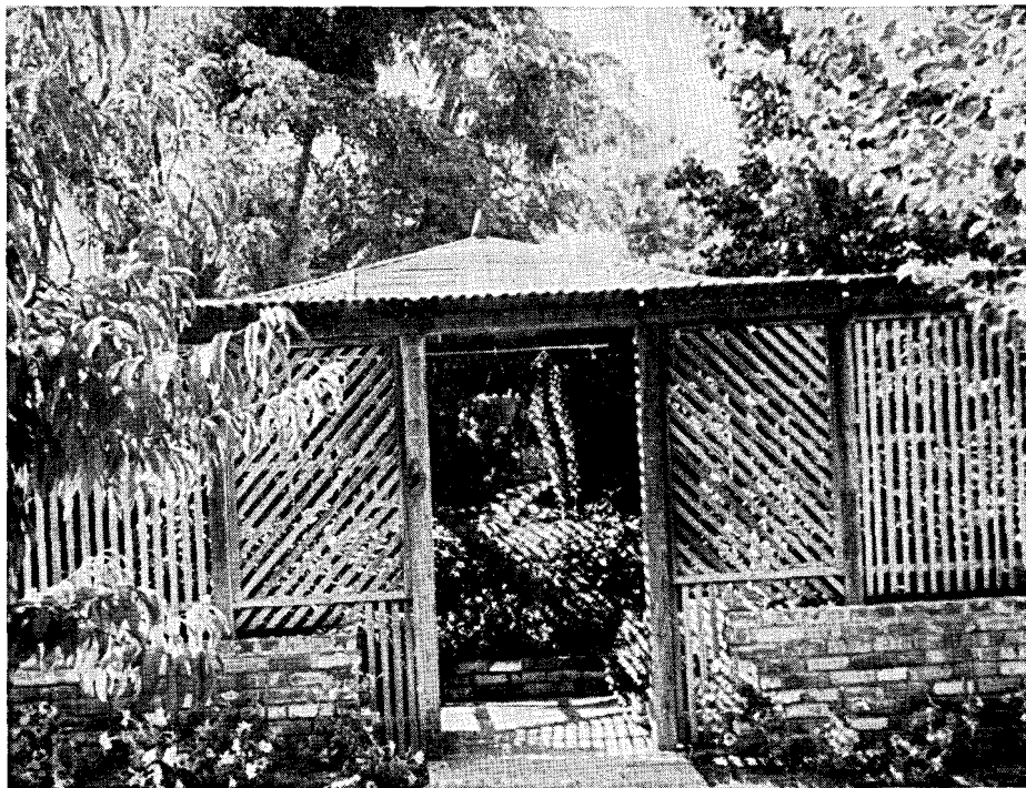
NEWTON PRATT'S house, Sacramento, California, which enhances rather than detracts from the landscape.
