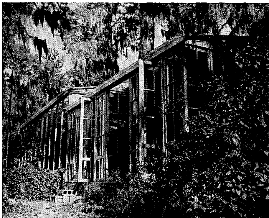
Exterior of greenhouse showing how it blends into setting
