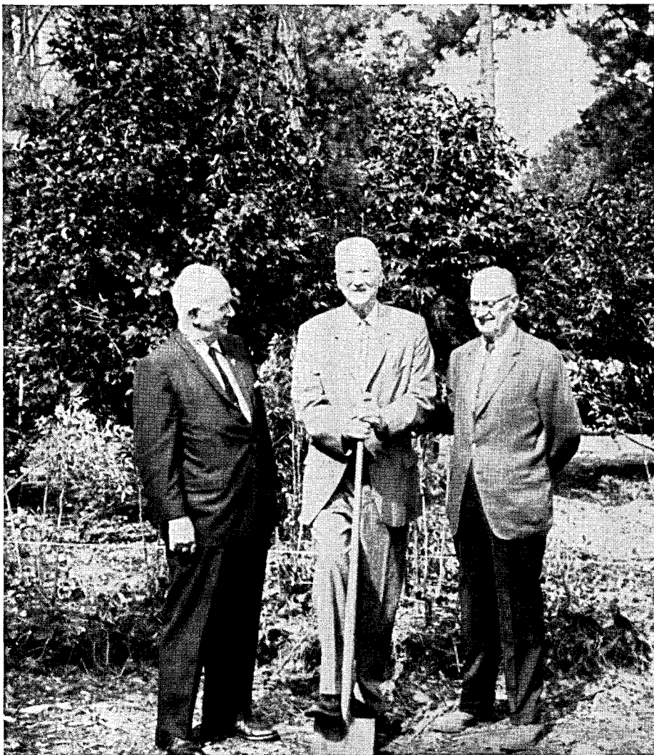
HEADQUARTERS GROUND BREAKING. On September 5 actual construction on our new Headquarters building at Masse Lane was started. Mr. Dave Strother who donated his famous Camellia garden and $37,000 toward its endowment turns the first shovelful of earth at the site. On his right is ACS Vice-President Payne H. Midyette, Chairman of the Endowment Fund Raising Committee, and on his left is Vice-President Terrell Weaver of the Building Committee. The contract specifies that the building be completed in 180 calendar days.
