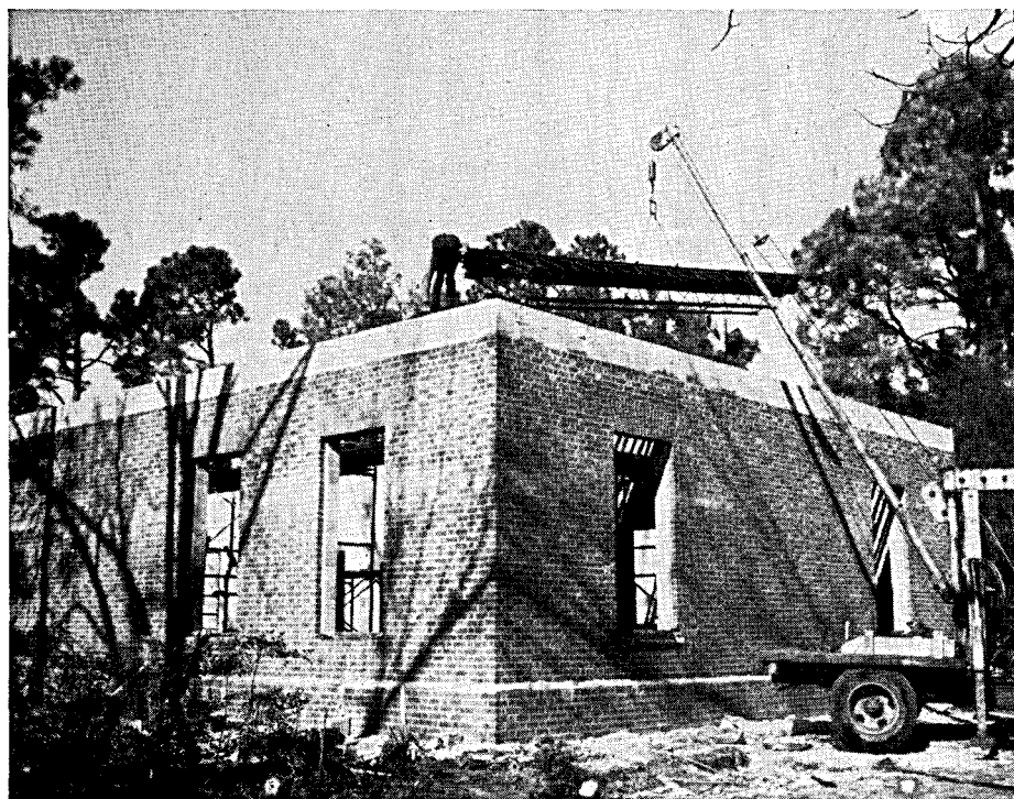
Progress on ACS Headquarters at Massee Lane December 4, 1967. Brickwork completed, steel girders to support concrete attic floor being lifted into place.
