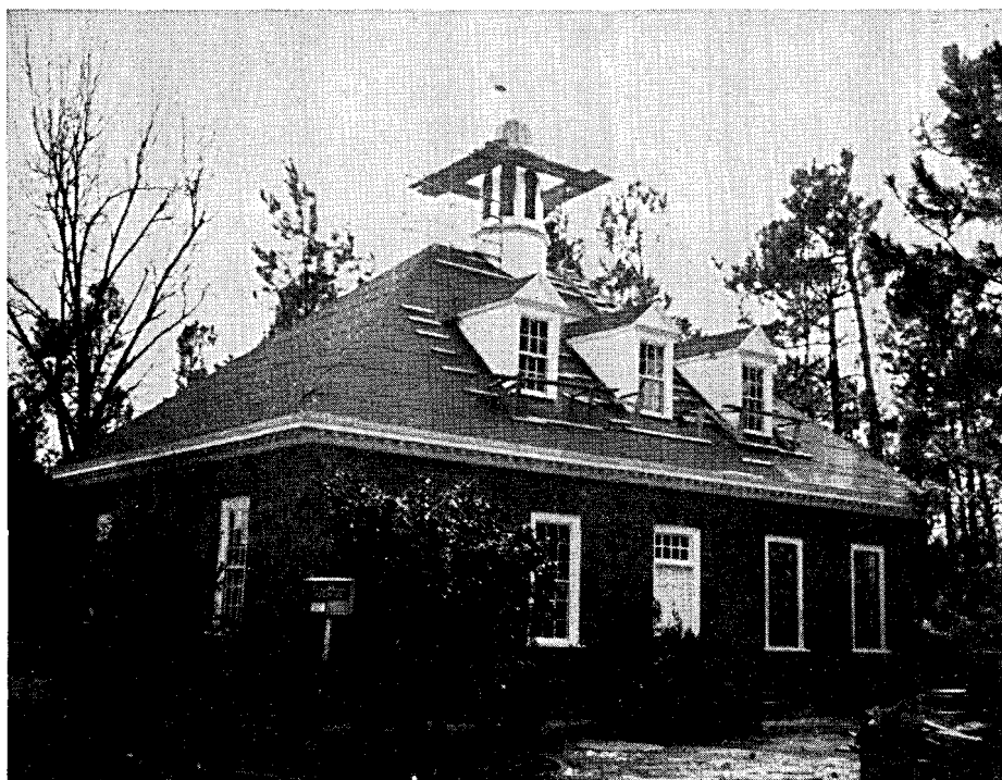
Exterior of ACS headquarters nears completion on March 2, 1968. Plastering completed. Contractor promises completion of interior by April 15th.
