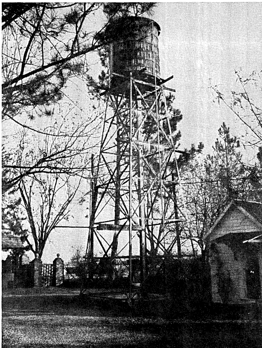
The old water tank tower near the entrance. Since we now have a new deep well elsewhere in the garden, this tank will be torn down. The two smaller wells at its base will be connected to a small pressure tank behind the pierced brick wall. The small office has been renovated and will be used as an office for the horticulturist when we can afford one. When we had a bid of $400 for the pressure tank and removal of the old tank, Mr. Strother offered to meet this expense.
