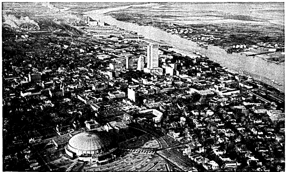
Panoramic view of Auditorium, our hotel-motel, historic section and the busy port of Mobile.
