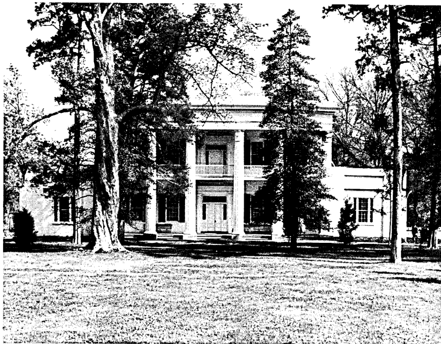
"Hermitage"—Home of Andrew Jackson (Photo Courtesy of Nashville Area Chamber of Commerce)
