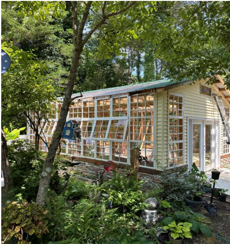
Roof was completed, brick facing covered the entire perimeter, and the front was completed. Decorative trim was installed to cover the hinges and gaps between the windows.
