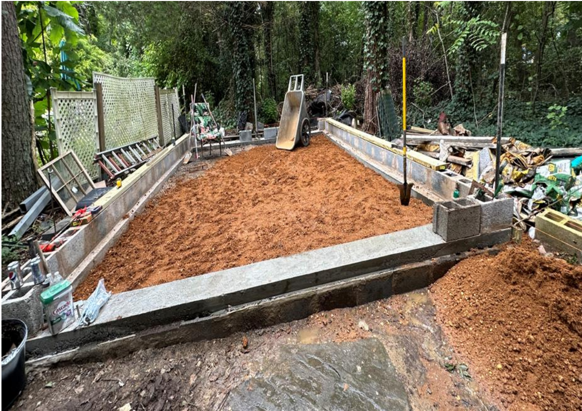
While the first row of the block wall was being completed all the way around, we brought in dirt fill to bring the floor up to level.
