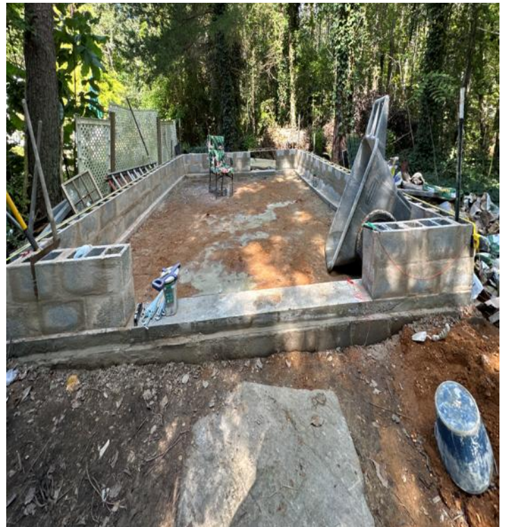
The second row of block was completed all the way around, with spaces left for the doors.
