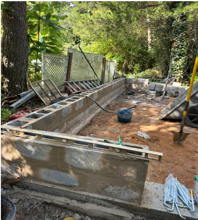
The second row of block was placed, making sure it was level and straight, and the block had staggered joints.
