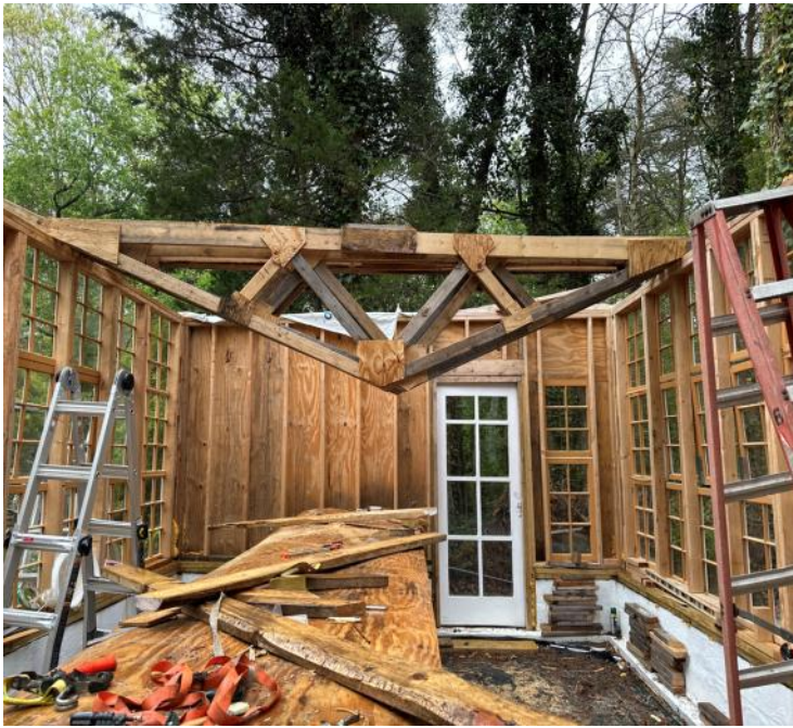
As each truss was constructed, it was hung upside down in place until all the trusses were completed and roof construction was ready to begin.
