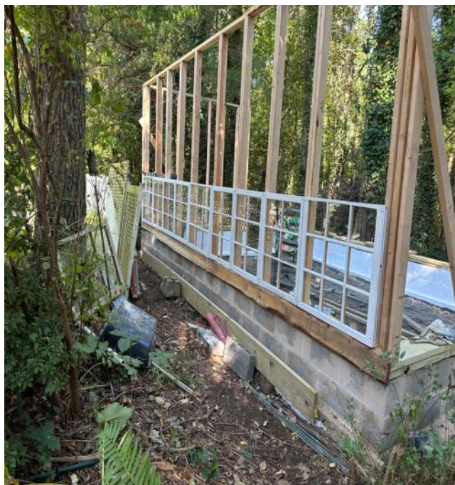
As the stud frames were completed on each side, we began attaching the windows that make up the walls. The bottom row of windows is fixed in place and they do not open.
