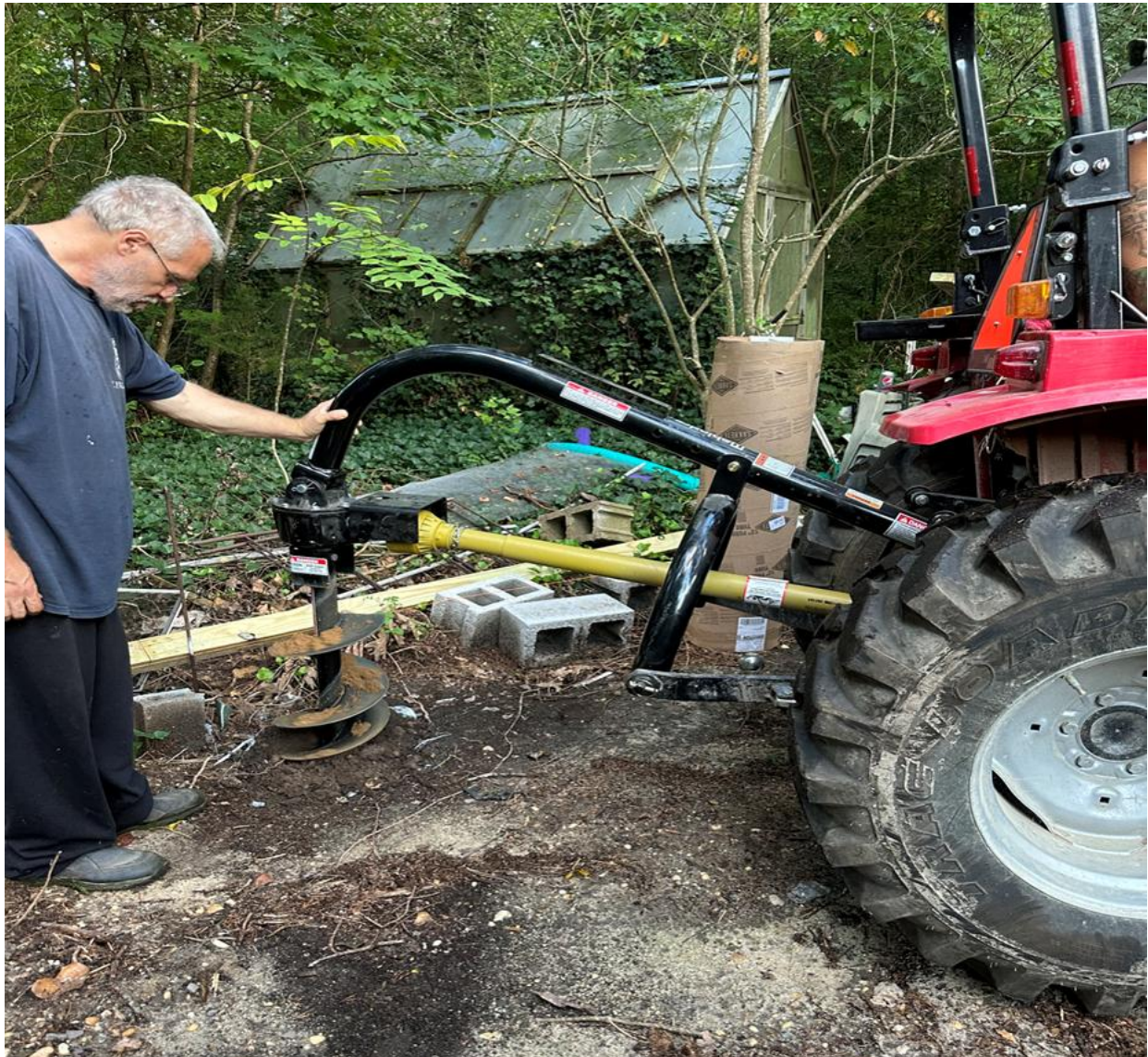
Placing the auger to dig out the footers; centering it underneath where the perimeter lines cross. Six footers were dug, each 24" deep.
