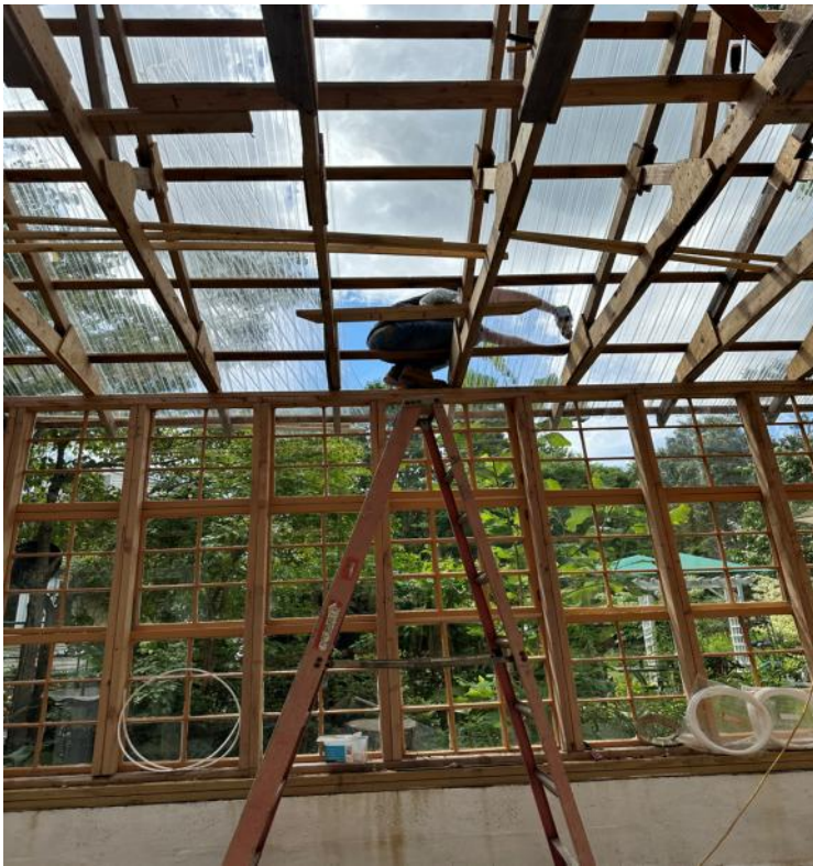
Fastening the roof panels to the cross beams for added support.
