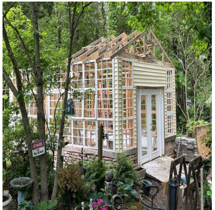
The trusses were flipped upright and fastened to the top of the window walls, then tied together with cross beams.
