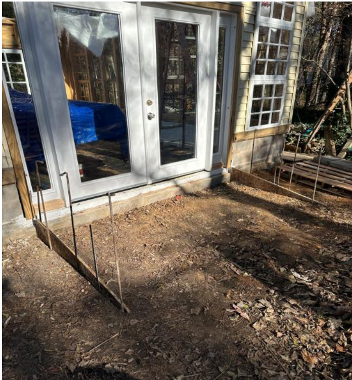
We constructed wooden wedge forms for the ramp and temporarily fixed them with rebar.
