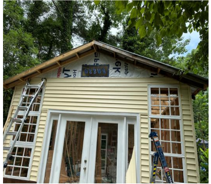
When the roof was completed, the stained-glass sign was installed and an eave was added to the front of the building.
