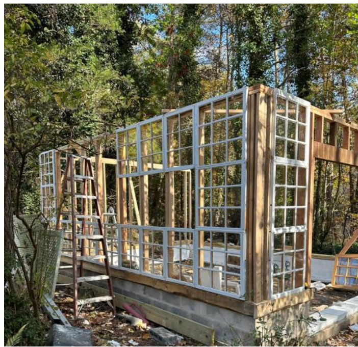
The top row of windows and the corner windows are also fixed and do not open, so they are mounted next.
