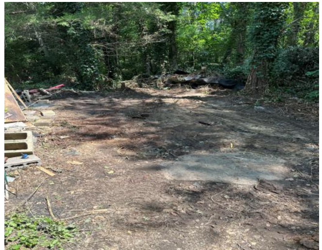
Area where the old shed used to be, cleared of the shed and brush, ready for the initial layout of the new greenhouse floor plan to see how big it could be and if more brush or trees need removal.
