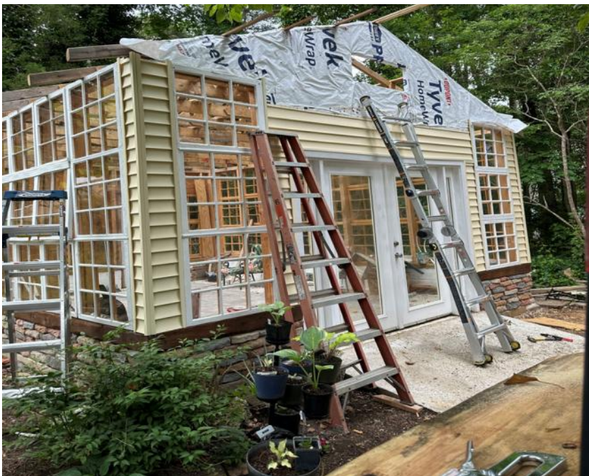
As each truss was constructed, it was hung upside down in place until all the trusses were completed and roof construction was ready to begin.
