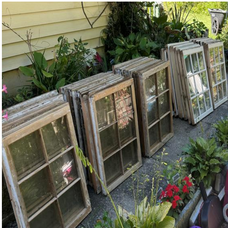
Reclaimed windows that have been stripped, sanded, repaired, and cut to the correct size, waiting to be coated with outdoor paint.
