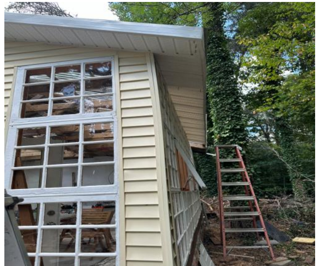
Soffits were installed to hide the gaps in the overhang of the roof, and to keep birds and pollinators from becoming trapped.
