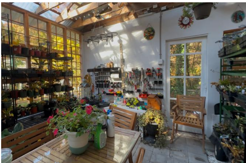
Back inside completed with benches and shelves installed; began filling with plants for the winter.
