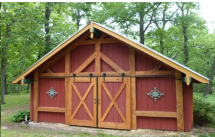
The Timber Frame façade on The Shop.
