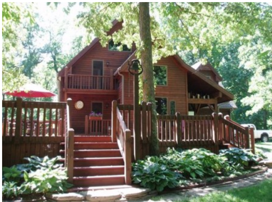
The greatest project of Phil's life- the multi-story timber frame home that he constructed by himself.
