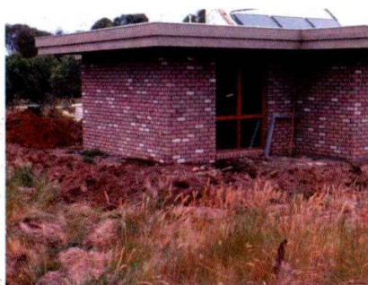
The mess when the house was being built
