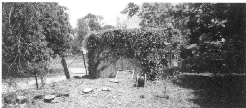
Work in progress, Oct 2003. Gone are the wattles, japonica, ivy and periwinkle. Tank covered in dead ivy. See the change on page 184.
