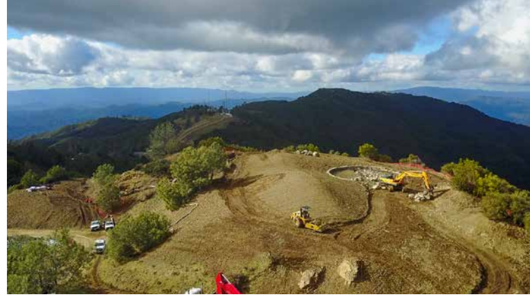
An aerial view of the Mount Umunhum construction site as the summit was being rebuilt.
