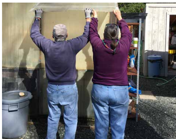
Jean and David in action, repairing a greenhouse roof at the nursery.
