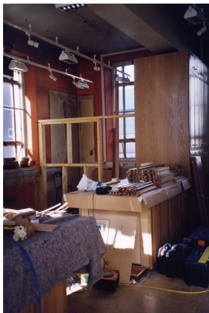
Work in progress at the far end of OXF (July 2003, photograph: S.K. Marner).
