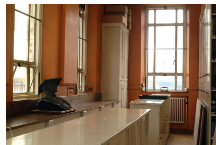
Far end of OXF before refurbishment (February 2003, photograph: J. Baker).
